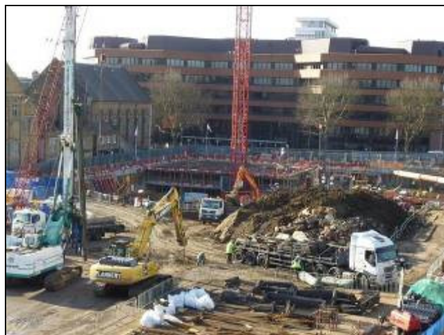
The Dickens Yard basement taking shape
