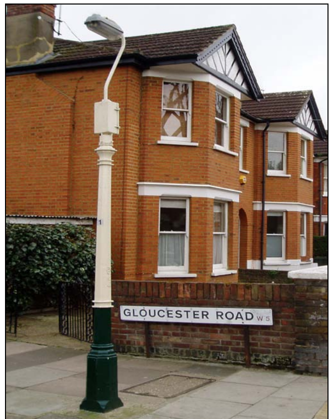
One of the original gas lighting columns (now with a modern light attachment).
