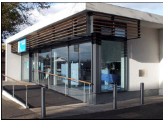
The new front elevation of Northfields library.
